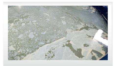
Figure 18. Appearance of floating grease in grease trap.
