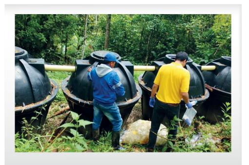
Figure 19. Septic tanks installed in the department of Cauca.
