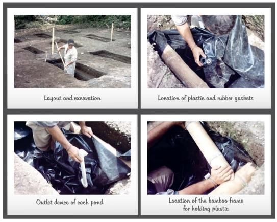
Figure 32. Construction of horizontal subsurface flow wetlands (Source: Rodríguez, 2009).
