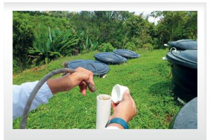
Figure 25. Purging of the system for sludge removal.
