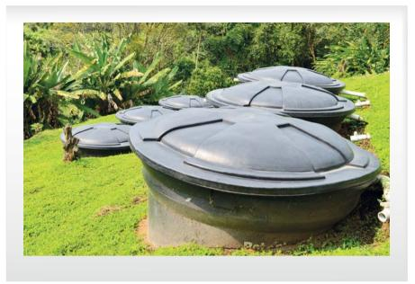
Figure 28. Half-buried anaerobic filters.
