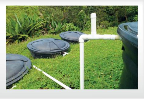
Figure 24. Coupling of inverted-siphon pipeline or device for sludge removal.
