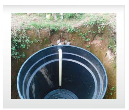
Figure 22. Pipe inside the septic tank for sludge removal.
