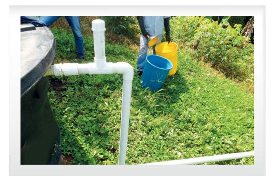
Figure 23. External pipeline or device for sludge removal.
