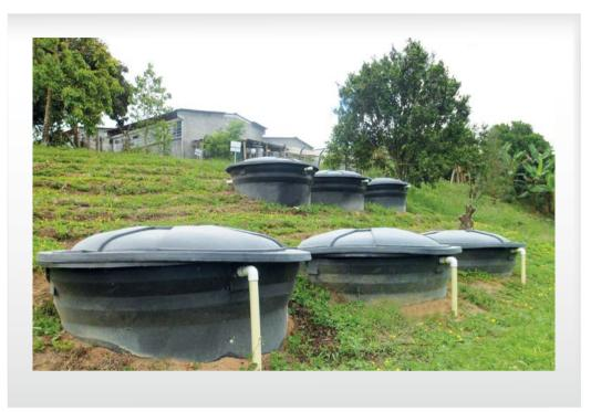
Figure 21. Half-buried septic tanks.
