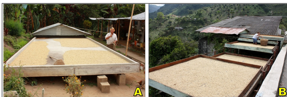
Figure 3. Typical small-scale movable drying structures: (A) Sliding-roof platform (casa-elda) and (B) multi-tier sliding tray system. Photographs taken by the authors; images are provided as representative examples of commonly used small-scale drying systems.
